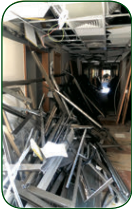
Damages resulted from the blast
