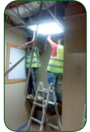
Today: Re-constructing Rosaire's Hospital Eye Center
