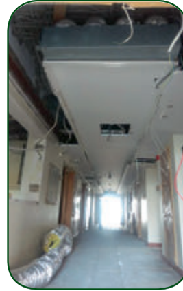
Today: Re-constructing Rosaire's Hospital Eye Center
